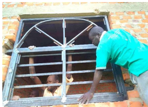
Window installation at Ojeburun Lutheran Church
